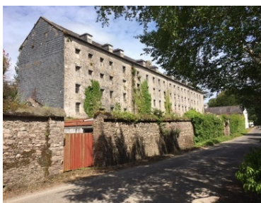
Main mill building with slate hung south gable
