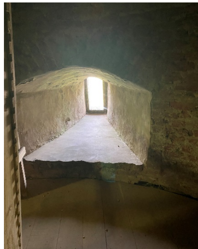
Arrowslit exhibiting wall thickness and oblique angle of cutaway to increase the defender's field of vision
