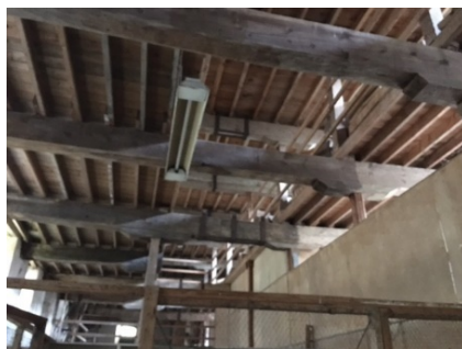
Detail of large transverse baulks
