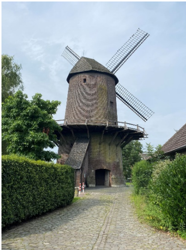
East side - ground floor entrance and external stairs to second floor
