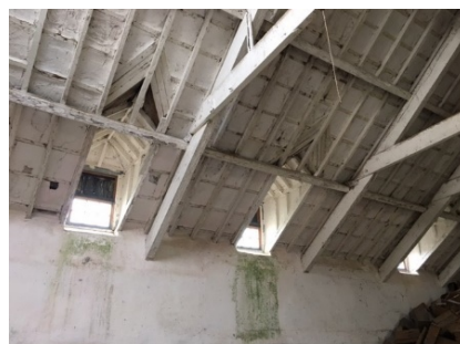
Detail of inner roof and dormers
