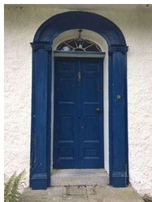
Wages office reinforced door with gun hole in centerboard
