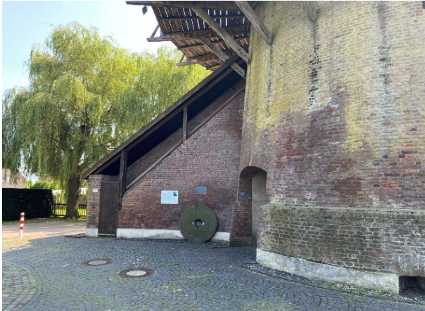
External stairs to main milling floor
