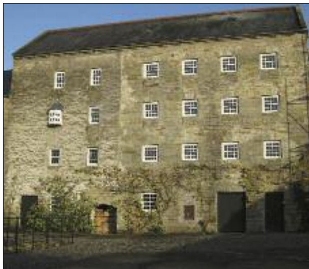
Fancroft Mill from the mill yard, wheel visible in bottom centre opening.
