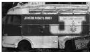
An old Johnston Mooney & O'Brien Electric Van at Dromod. Photo by S.Bourke.
